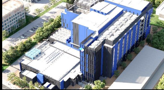
Macquarie Park Data Centre Campus IC2, IC3 East IC3 SuperWest
